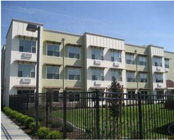
Figure 10: Photo of multi-storied modern apartment building
